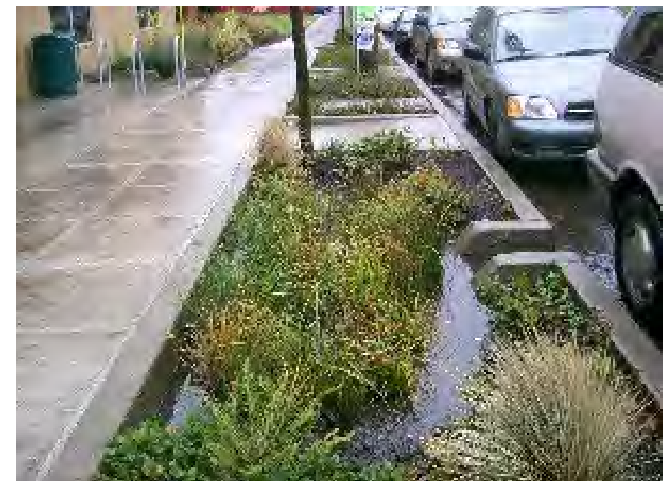
Swales along the edges of surface parking areas absorb vehicular run-off that would otherwise end up in the storm water and river systems.
