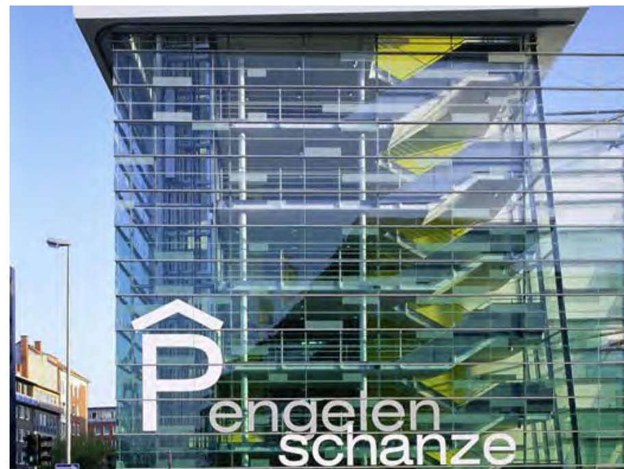
Well designed parking structures are attractive, centrally located and accentuate the context of the street like this one in Munster, Germany. Photo: W. Huthmacher
