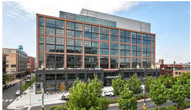
Mechanical penthouses should be screened or incorporated through building design
