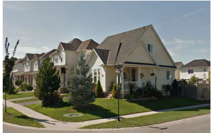
Dwellings should be sited and articulated to address all street frontages / Stowe Terrace
