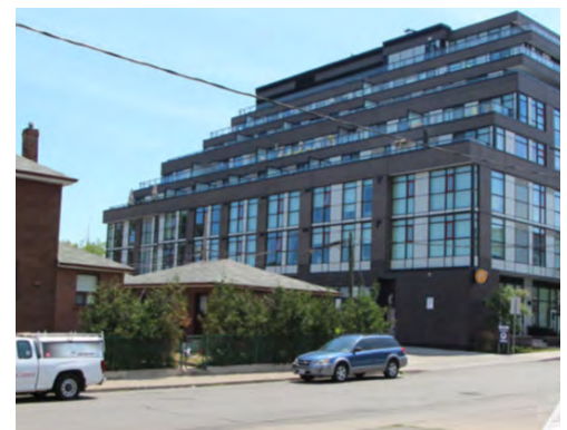
Transition to low-rise should be accommodated through building design, stepbacks, and buffering / Burlington, ON.
