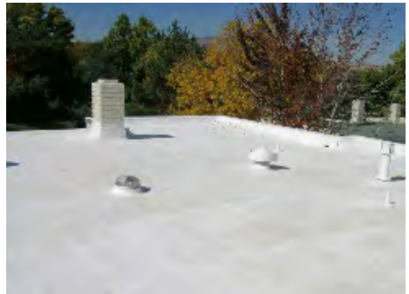
Light coloured roofs have a high solar reflectance, which reduces energy costs and the urban heat island effect.
