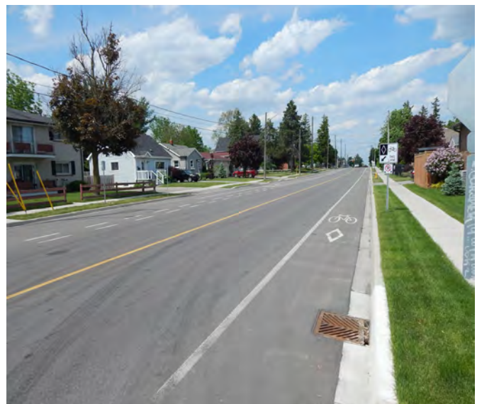
Accessible sidewalks should be provided on both sides of the street with adequate boulevard separation / Brantford, ON.
