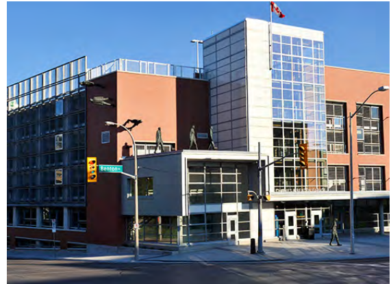
Parking structures should provide active at-grade uses and provide public art opportunities / Kitchener, ON.
