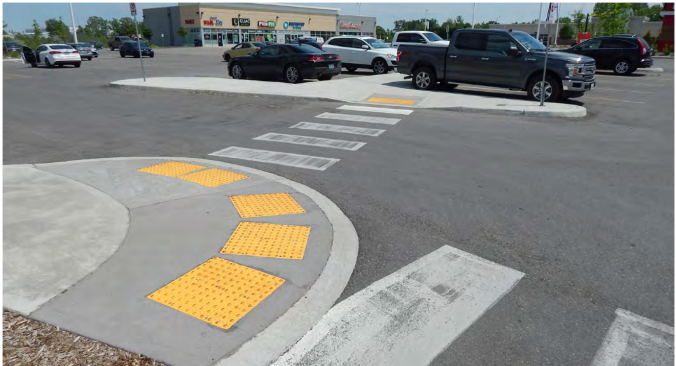
Tactile warning strips and slopes should be provided at pedestrian cross walks defined with distinct paving
