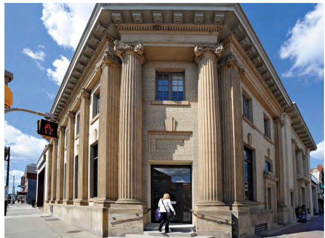
Corner buildings provide valuable opportunities to implement distinct architectural elements
