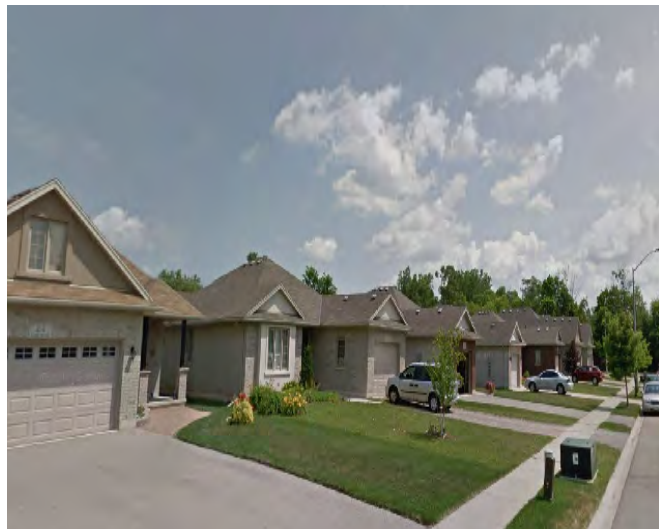
Controlled front yard setback variation provides visual interest on straight street blocks / Jamieson Ct.
