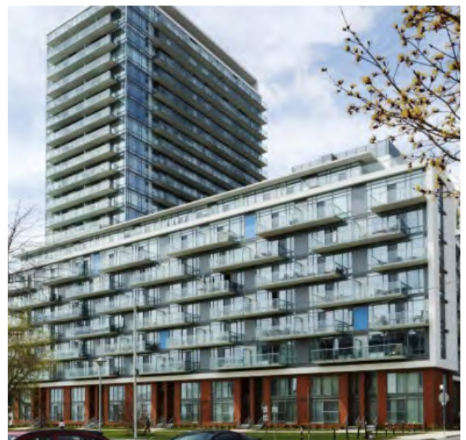
Buildings should include well designed and articulated podiums, middle sections, and tops / Toronto, ON.
