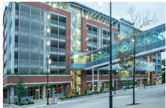
Above grade parking should be screened and at-grade parking should not be visible / St. Catharines, ON.
