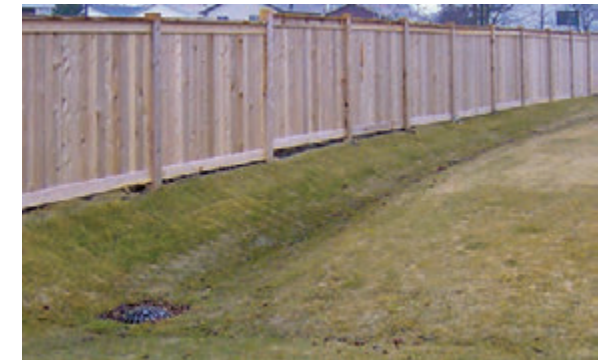
Rear-yard swales direct flows to a catch basin in this image. Rear-yard catch basins and swales shouldn't be covered or filled in with backyard sheds, fences or other structures, and rear-yard catch basins should be kept clear to reduce backyard flooding.
