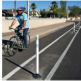
2) Painted Buffer with bollards,
