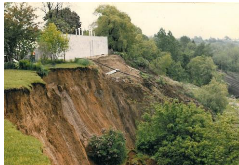
929 Colborne Street (East) after 1986 landslide
