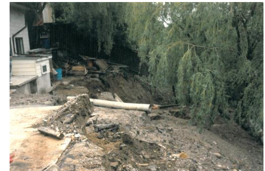
951 Colborne Street (East) after 1986 landslide
