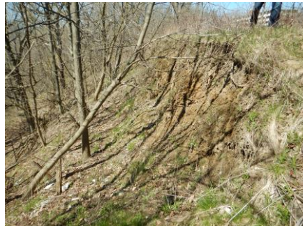
Slope monitoring in 2016, unstable slope evidence (left) and slumping near property line (right)
