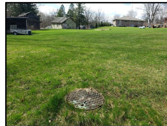
G. Looking Towards Peartree Court at Manhole 14
