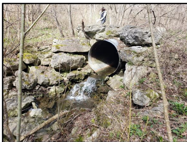
E. Existing Crossing over Combined Storm Outfall Channel
