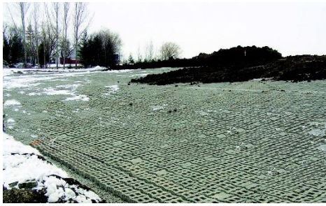
Figure 4-4: Example of Vegetated Concrete Block Installation (Nilex, 2022).
