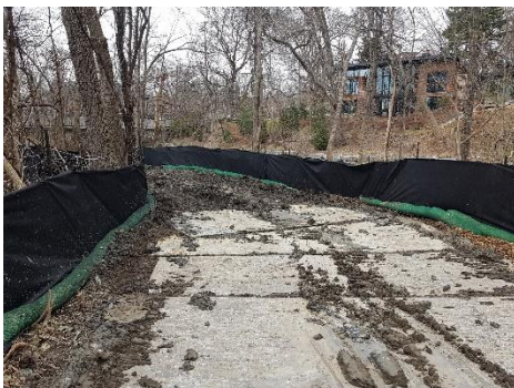
Figure 4-2: Example of Temporary Wood Matting with ESC Fencing.
