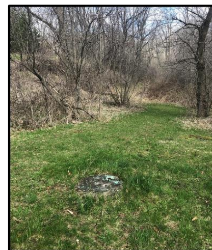
F. Looking Towards Wooded Valley Corridor at Manhole 14
