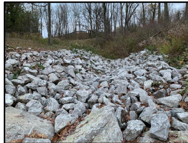
C. Emergency Back Stabilization Measures to Protect Exposed Sanitary Sewer (2019)
