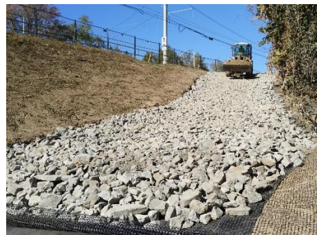
Figure 4-3: Example of Rock Geogrid Access Route.
