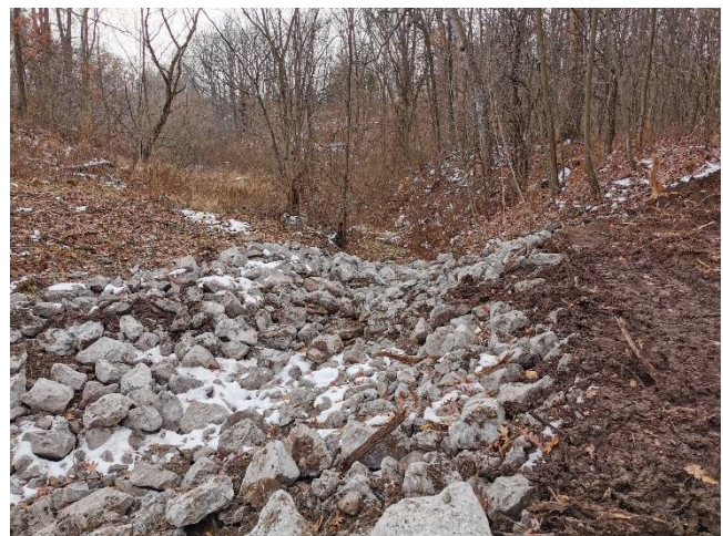
Figure 2-2: Sanitary Sewer Protect with Riprap Cover (Post-Repair, 2019)
