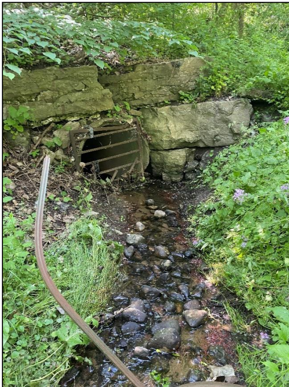
Figure 3-10: Culvert at Downstream Extent.
