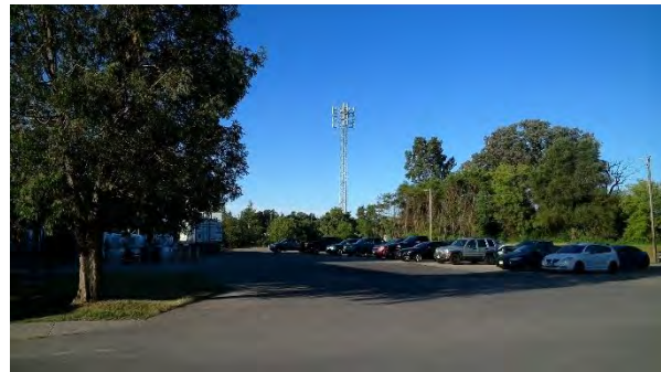
Photo 4. Telecommunications tower which contains an active Osprey nest (June 11, 2018).
