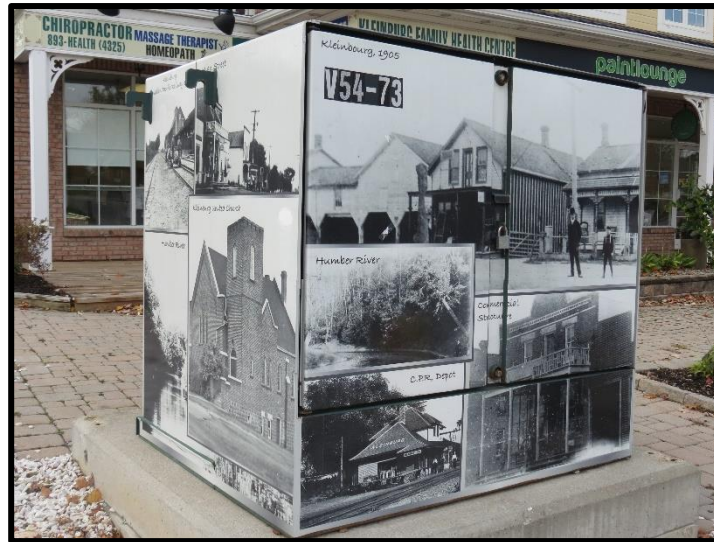
Plate 1: Electrical Box within Kleinburg Heritage Conservation District, Islington Avenue (ARA 2019)
