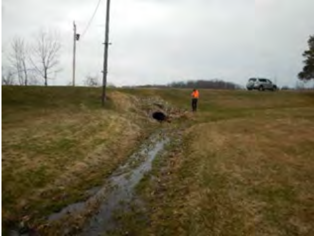
CAPTION: Downstream view to Golf Road culvert.
