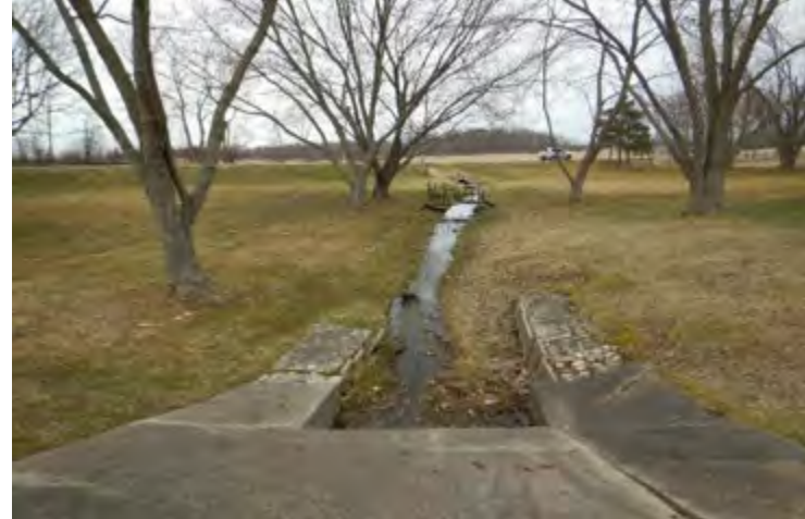
CAPTION: Downstream view towards Golf Road from landowner pedestrian bridge.
