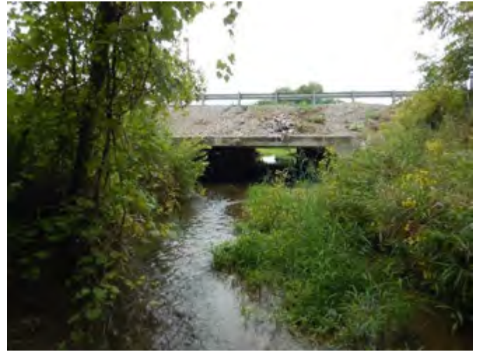
Photo 2: Road crossing culvert at upstream limit of reach
