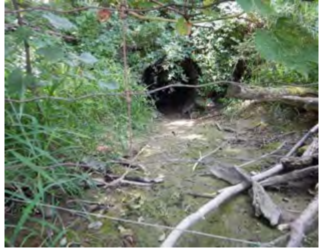
Photo 2: Culvert under trail (Id Karek Road)
