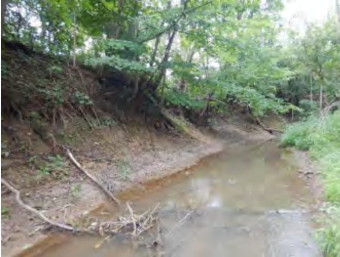
Photo 1: Bank scour, exposed roots, leaning trees
