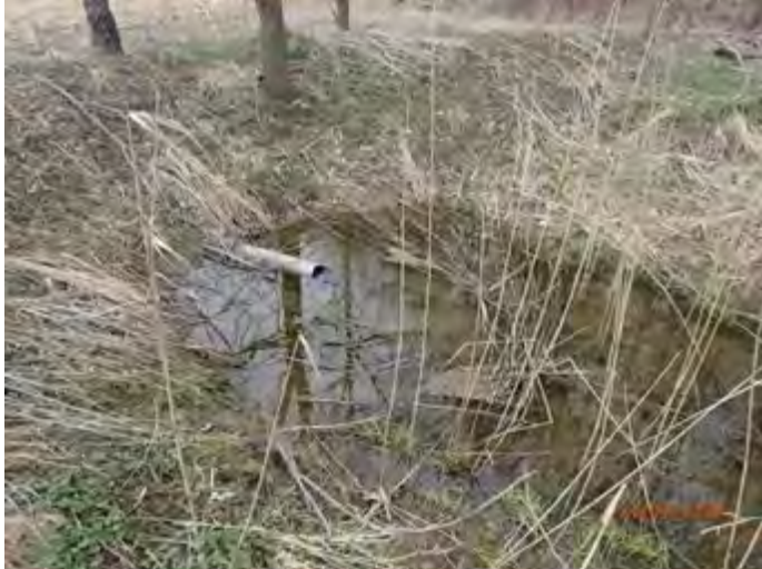
CAPTION: Outlet pool at upstream limit of drainage feature.
