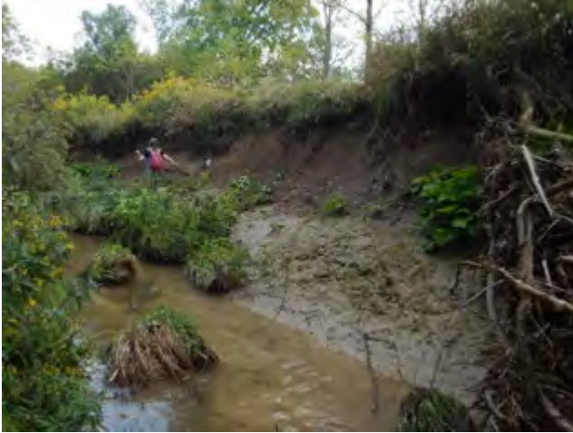
Photo 1: Scoured banks and cantilever bank failure blocks in channel
