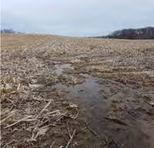
CAPTION: Standing water through drainage feature.
