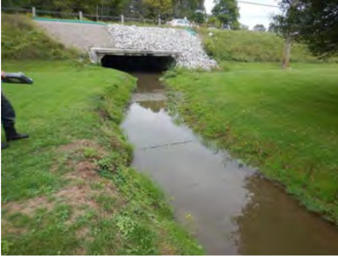
Photo 1: Road crossing culvert at downstream limit of reach.
