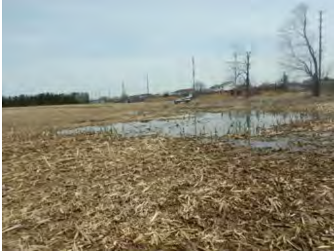
CAPTION: Downstream limit of feature – pooling of water in depression. Site visit #1 – April 2018
