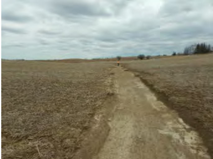
CAPTION: Downstream view – wide swale feature. Site visit #1 – April 2018
