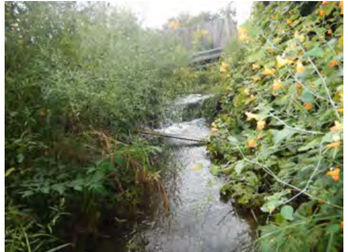
Photo 2: Constructed knickpoint in channel (0.5 m)
