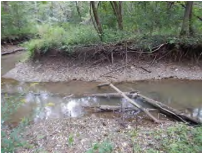
Photo 1: Bank scour at inside of meander bend
