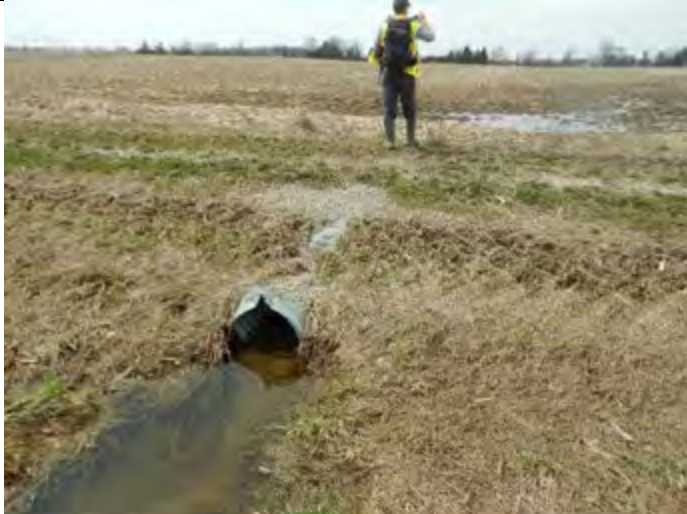
CAPTION: Upstream view of feature through private culvert crossing. Site visit #1 – April 2018
