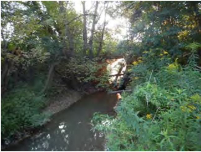
Photo 1: Road crossing culvert at downstream limit
