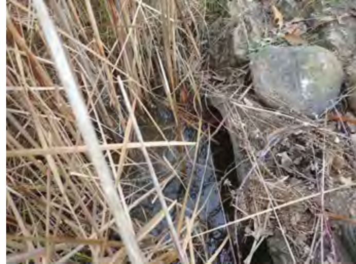
CAPTION: Feature piped through culvert under private laneway. Site visit #1 – November 2018
