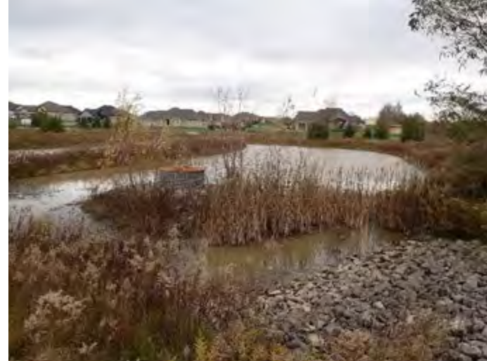
CAPTION: Stormwater pond located at upstream limit of feature. Site visit #1 – November 2018
