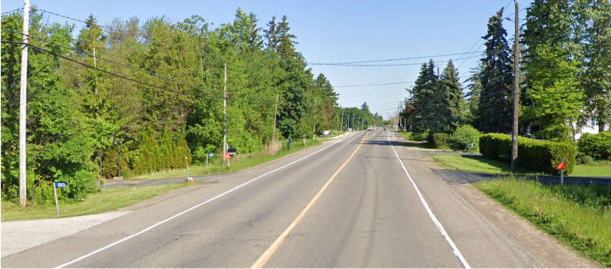
Figure 3-14: Paved Shoulders – Centre Road Waterdown, ON
