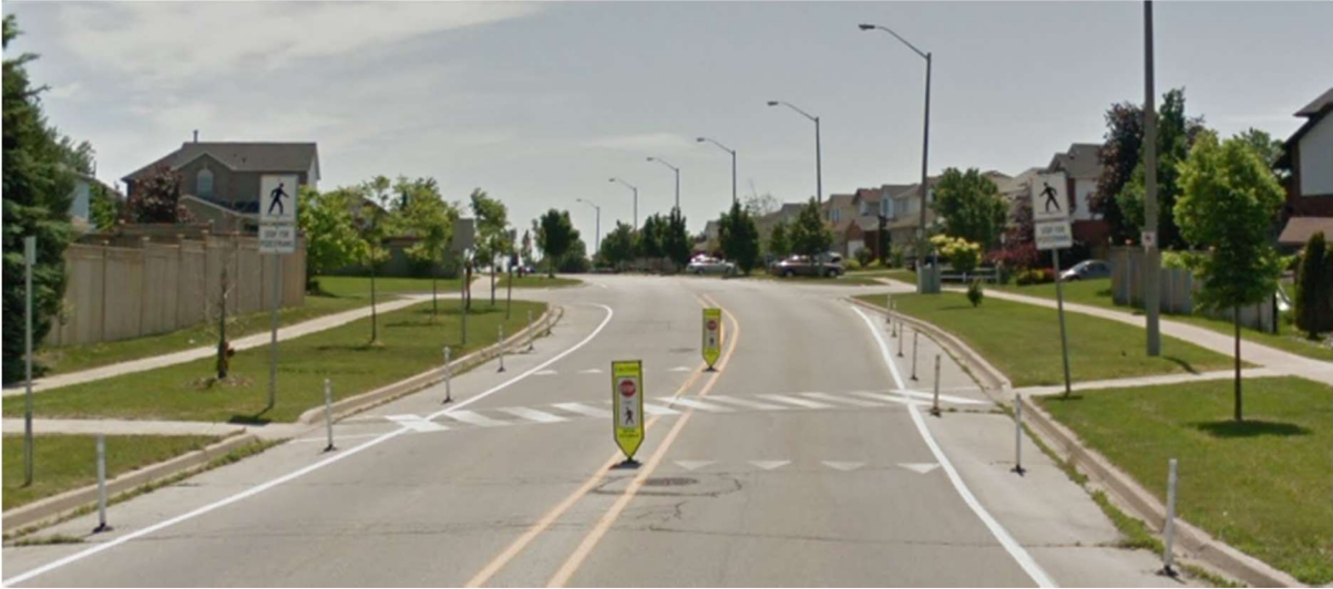
Figure 3-10: Pedestrian Crossover – Hollybush Drive Waterdown, ON
