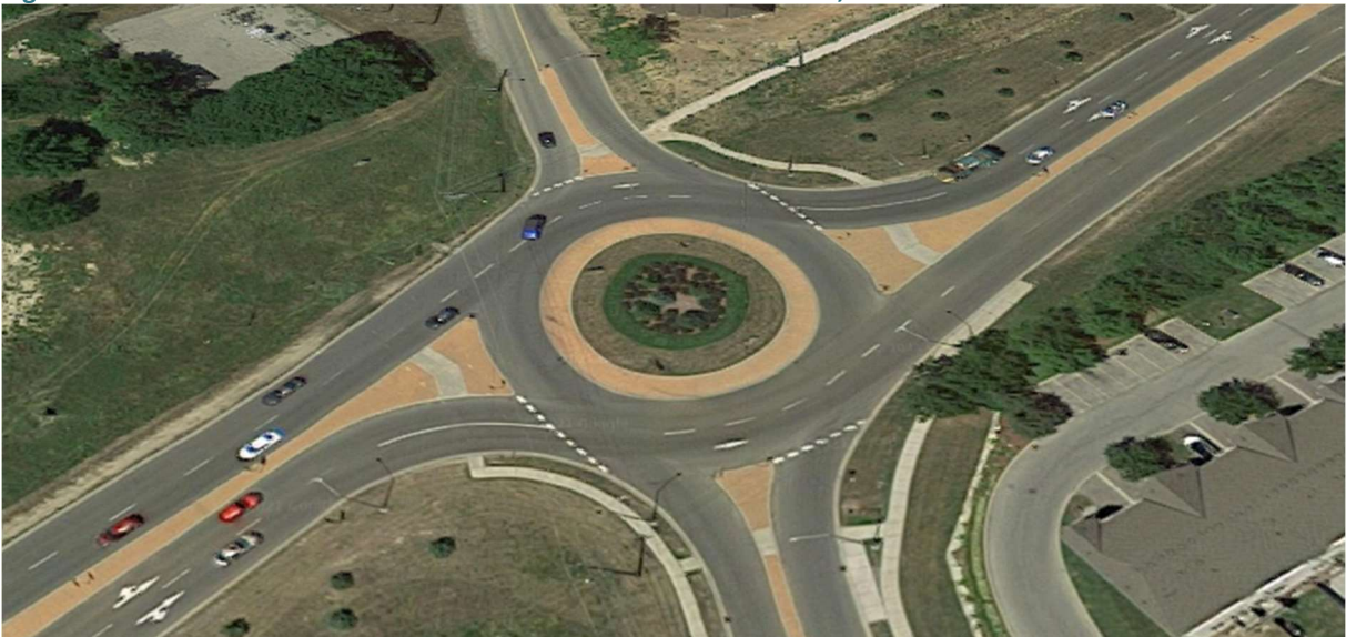
Figure 3-1: Roundabout - Wilson Street and Shaver Road in Ancaster, ON
