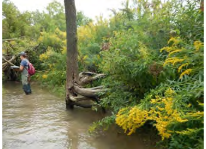
Photo 2: Exposed roots and tree within channel shows evidence of widening / migration
