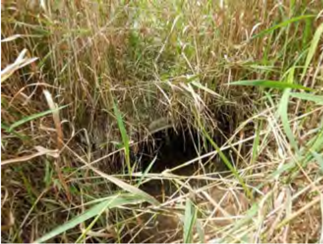
Photo 1: Tractor crossing culvert (0.5 m dia.)
