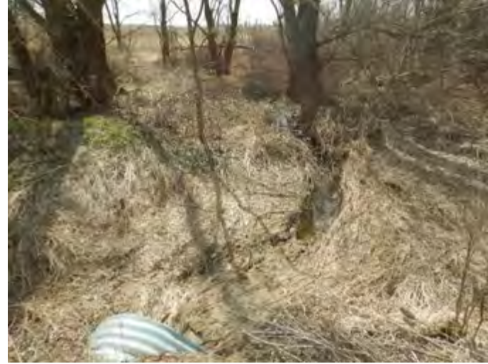
CAPTION: Upstream view – feature through culvert under driveway. Site visit #1 – April 2018
