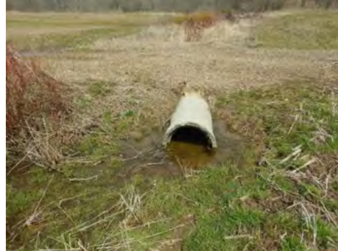
CAPTION: Concrete culvert under agricultural/private crossing. Site visit #1 – April 2018
