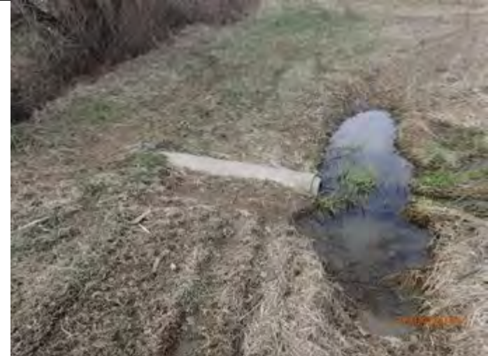
CAPTION: Feature at downstream limit of accessible properties; culvert through fence line. Site visit #1 – April 2018
