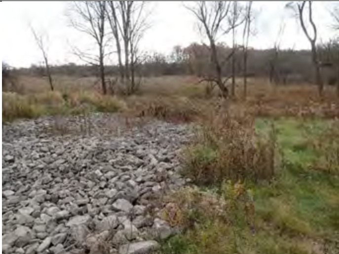
CAPTION: Riprap lined outlet to drainage feature. Site visit #1 – November 2018
