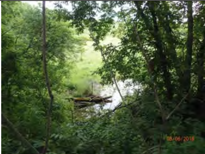
CAPTION: Water pooled upstream of culvert under private crossing. Site visit #1 – June 2018
