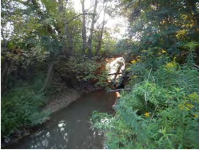
Photo 1: Road crossing culvert at downstream limit
