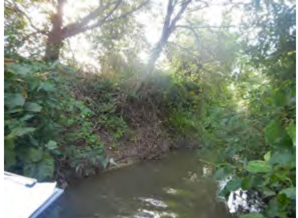
Photo 2: Bank erosion; exposed roots
