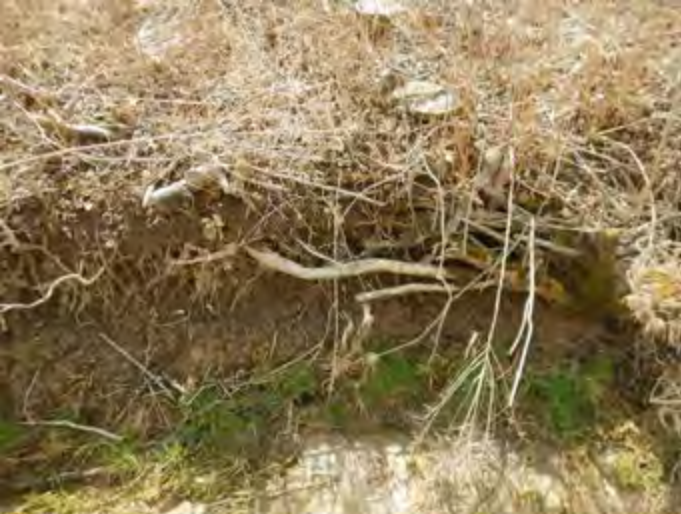
CAPTION: Erosion along feature; exposed roots and undercutting Site visit #1 – April 2018
