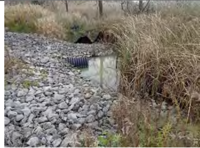
CAPTION: Outlet to drainage feature. Site visit #1 – November 2018
