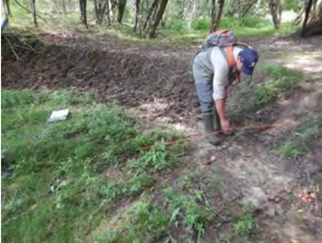
Photo 1: Channel cross-section; scour on outside bank
