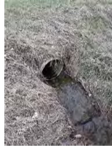
CAPTION: Outlet from Golf Road to drainage feature.
