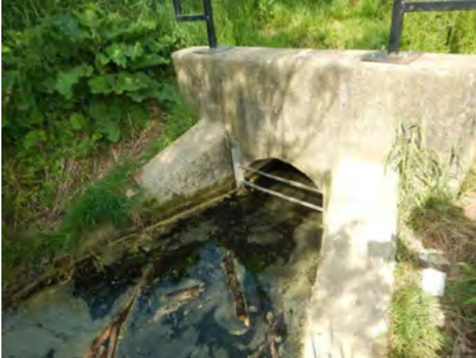
CAPTION: Grated outfall at upstream limit of feature. Site visit #1 – June 2018
