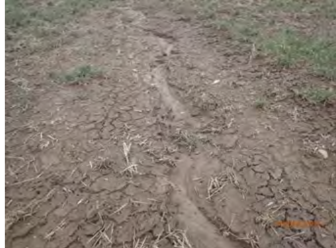
CAPTION: Some rill formation in exposed soil material. Site visit #1 – April 2018
