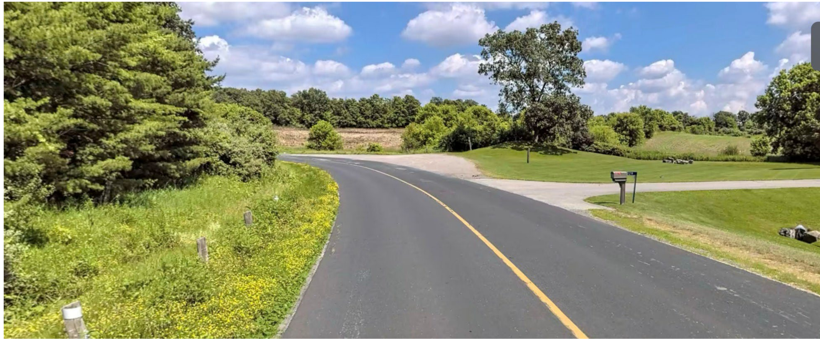
FIGURE 02: Photograph of Existing Roadway (Looking East)
