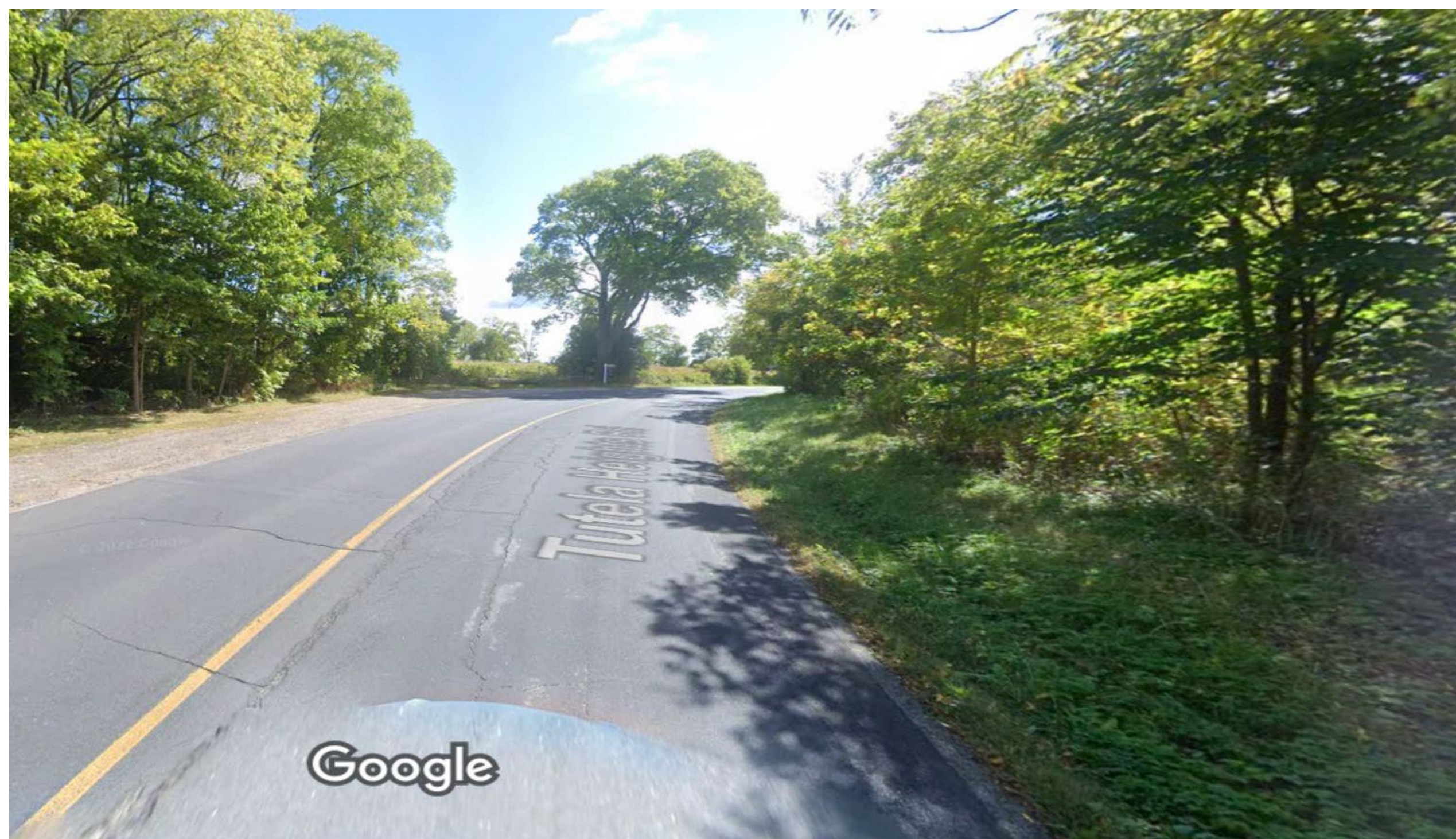
FIGURE 05: Photograph of Existing Roadway (Looking East)
