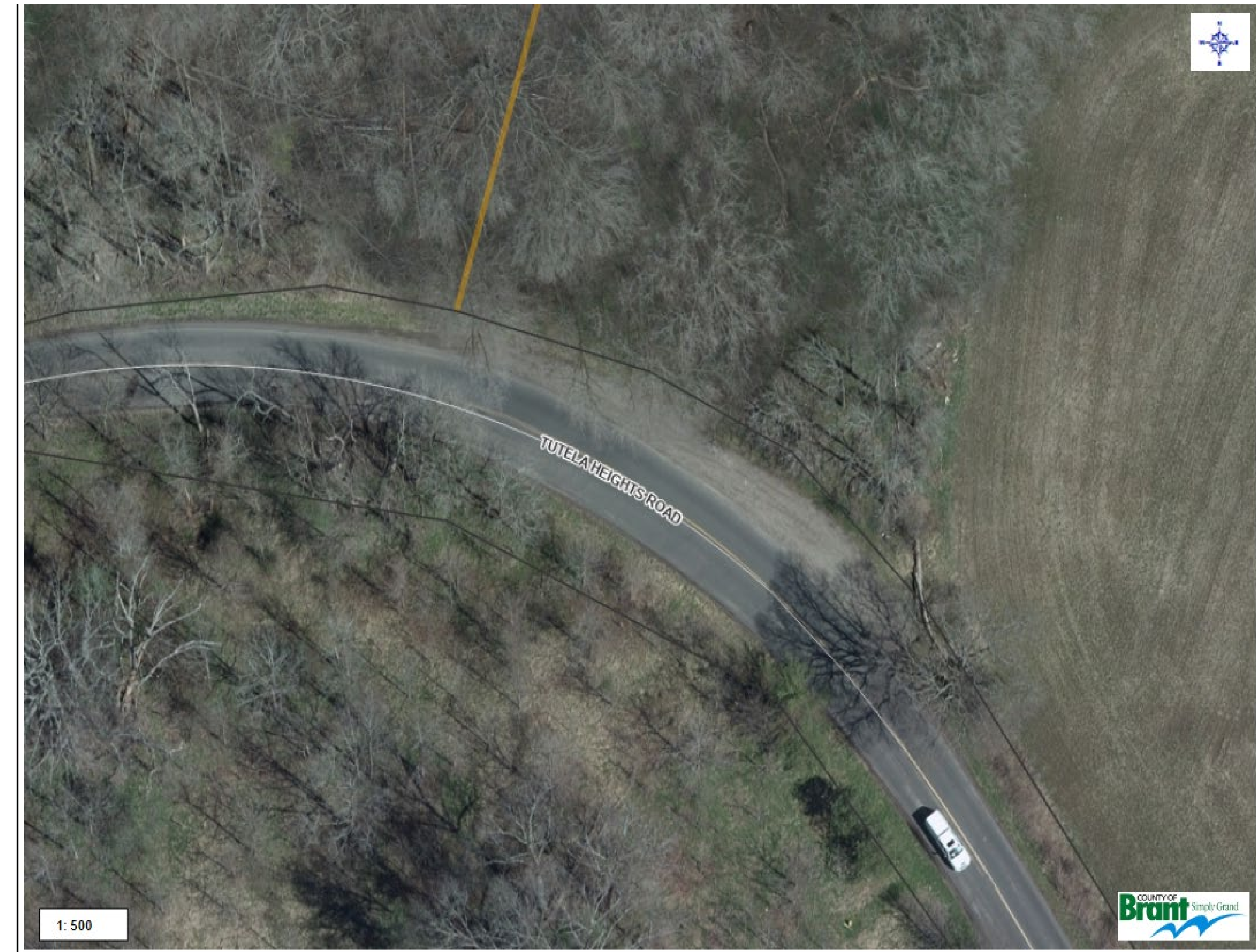
FIGURE 10: Photograph of Existing Roadway Proposed Hammerhead Location (Plan View)
