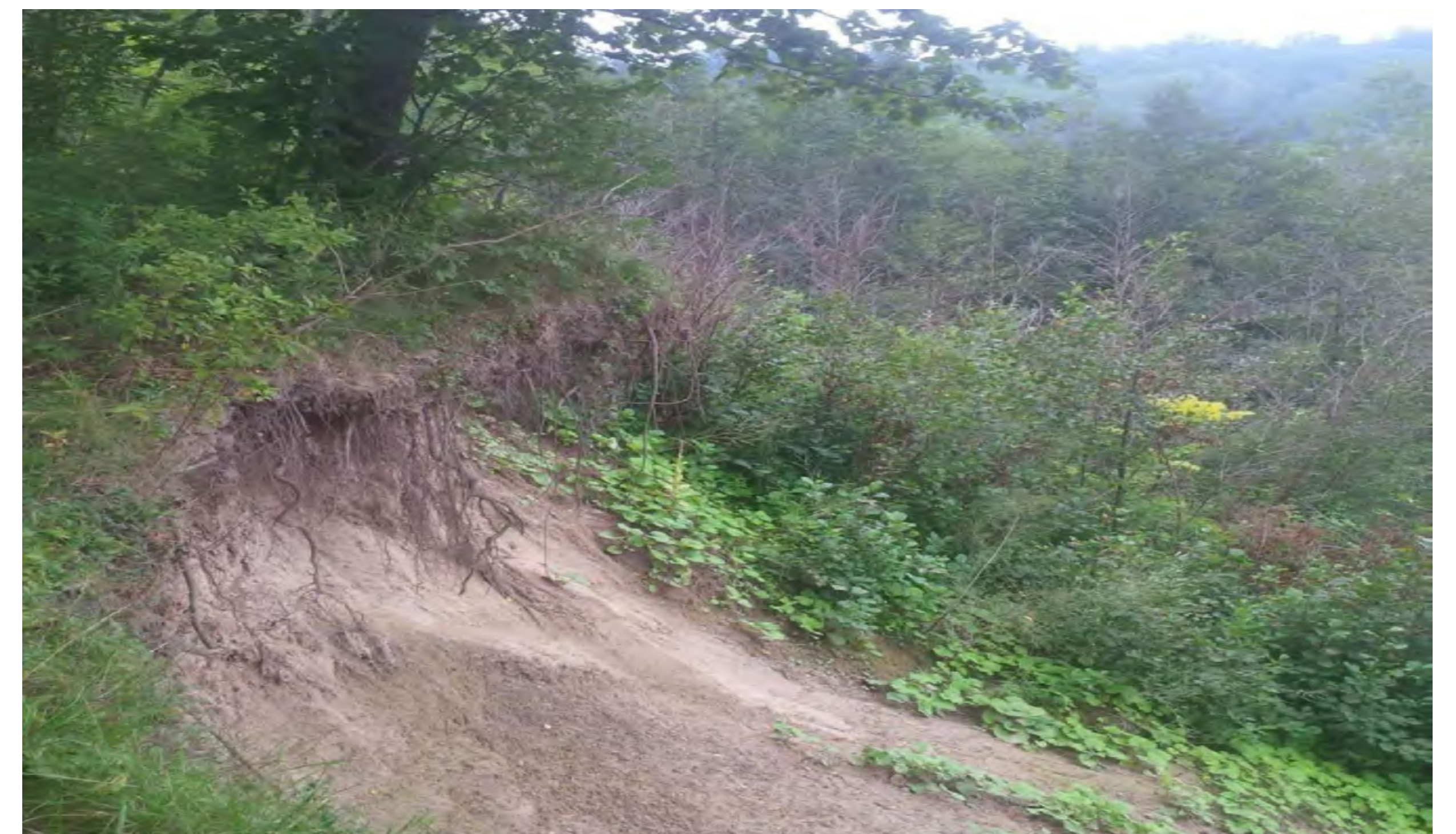
FIGURE 06: Photograph of Slope Failure
