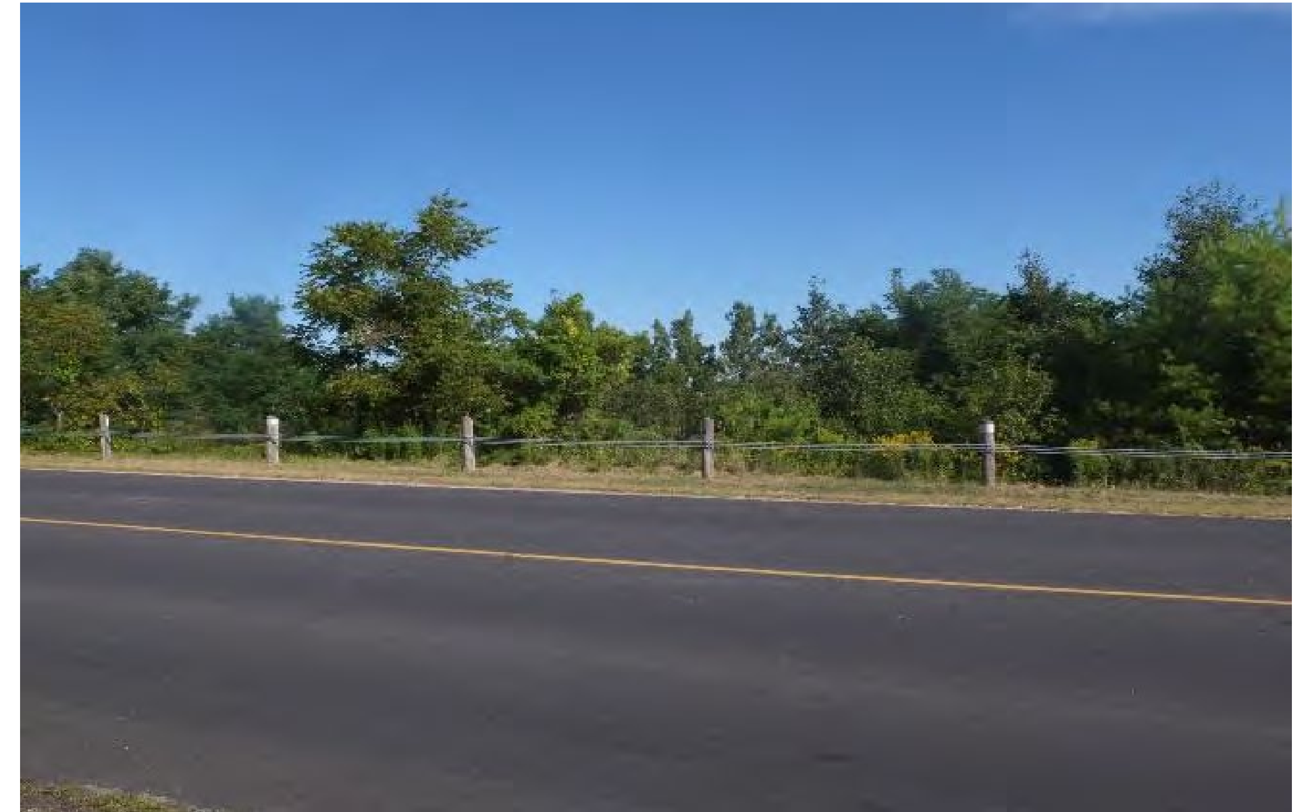
FIGURE 04: Photograph of Existing Roadway (Looking Towards Slope Concern)
